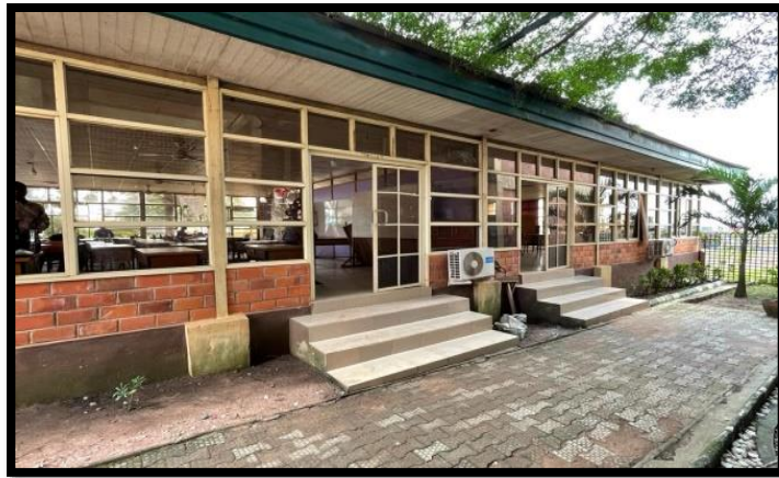
Plate 8: Large Double Swing Casement Doors at Glasshouse. Source: Researcher's Fieldwork, 2022
